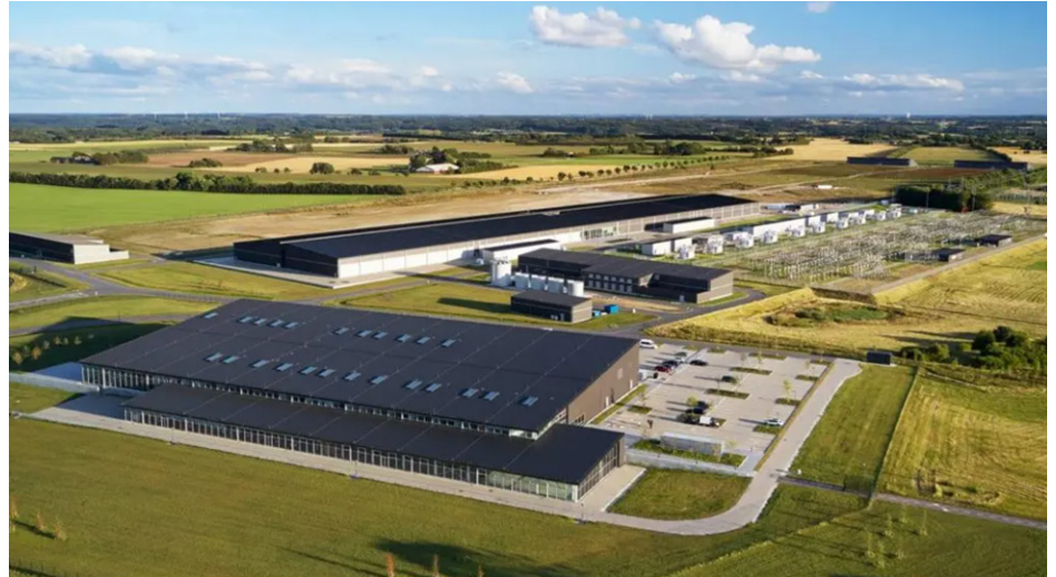
IMAGE 2: One of Apple’s data centers located in Denmark.
